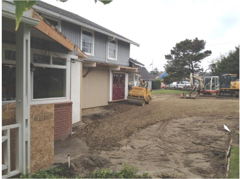
A corner of the main dining room is removed, plus some sewer work is accomplished, all in preparation for foundation work.
