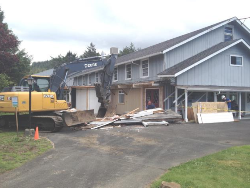
A corner of the main dining room is removed, plus some sewer work is accomplished, all in preparation for foundation work.
