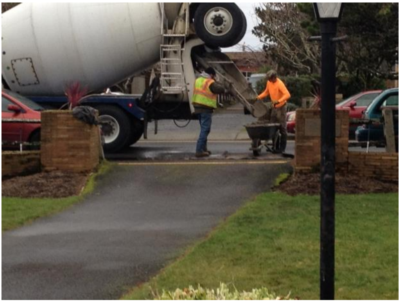
The tedious job of pouring a foundation under the old dining room where the corner has been modified.
